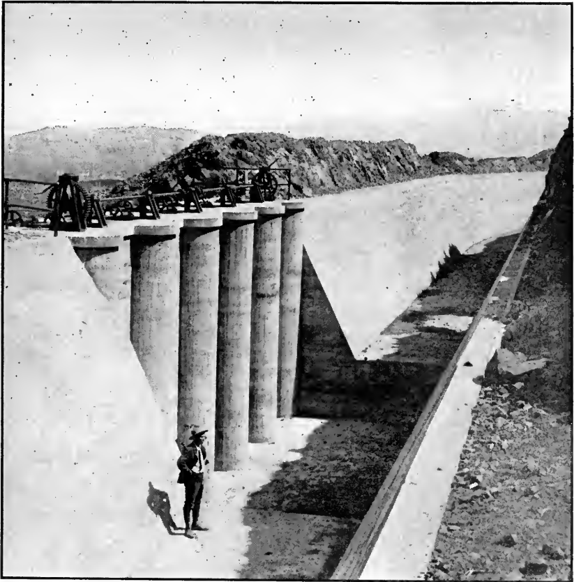
UP-STREAM FACE OF WASTE GATE, CANAL NO. 1, TRUCKEE-CARSON PROJECT
